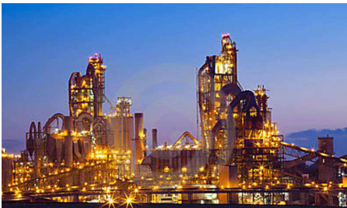
A modern petrochemical plant
